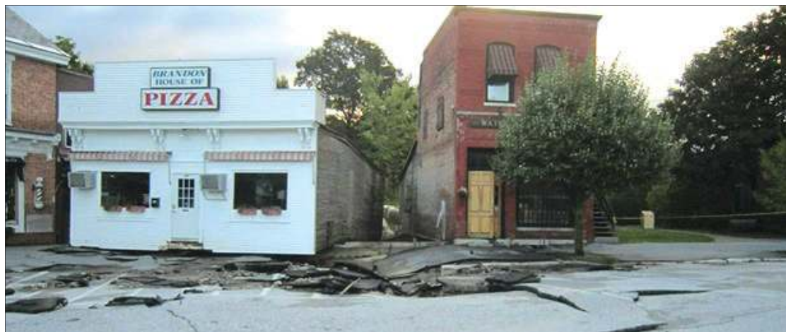
31 CENTER STREET remains intact while the former Brandon House of Pizza sits in the street in the aftermath of Tropical Storm Irene in 2011. The high-quality mortar used by mason Roscoe Sander likely preserved the brick building.
