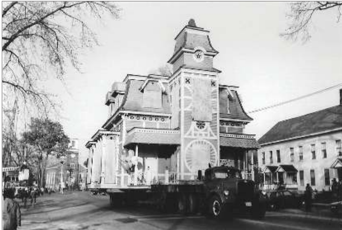
THE BIRD CAGE mansion en route through Conant Square. The Brandon Baptist Church is visible in the background. It would take several hours to move the mansion and its carriage house from its original location on Conant Square to its new home on a hill overlooking Wheeler Road.
