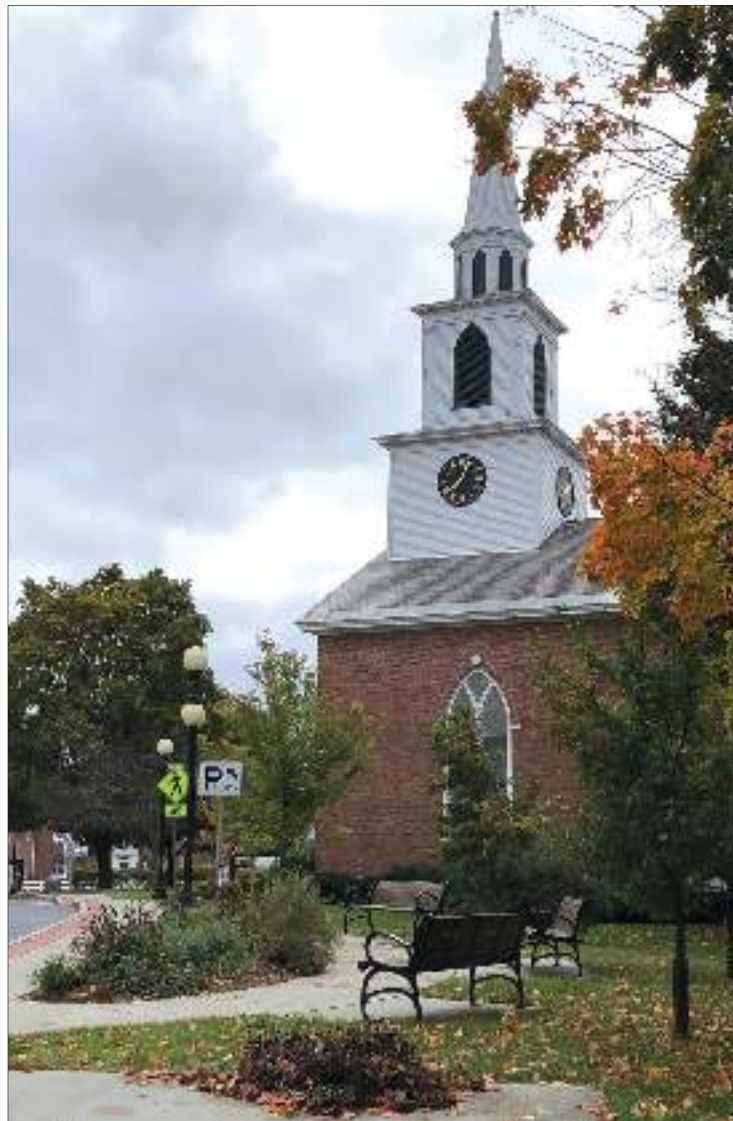
A VIEW OF the steeple and town clock on the Brandon Congregational Church. The brick church building dates to 1832. The clock was installed in the early 1890s. The clock and the steeple, both cherished Brandon landmarks, will require costly repairs.
