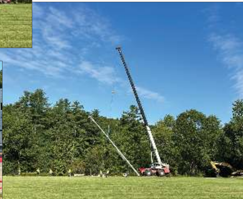
THE CREW THAT helped erect the light poles included Naylor & Breen, Markowski Excavating, and Benoit Electric. Each pole measured 80 feet long and weighed 10,000 lbs. The poles had to be raised by a crane and slid into prepared holes. Because of the wet ground, mats were laid to support the weight of the crane and protect the field. Photos by Steven Jupiter
