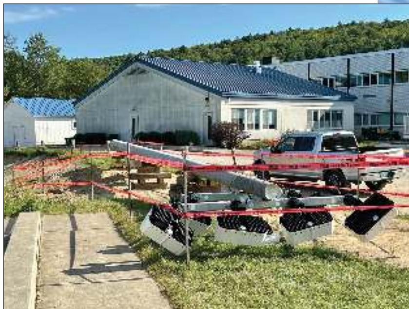
THE CREW THAT helped erect the light poles included Naylor & Breen, Markowski Excavating, and Benoit Electric. Each pole measured 80 feet long and weighed 10,000 lbs. The poles had to be raised by a crane and slid into prepared holes. Because of the wet ground, mats were laid to support the weight of the crane and protect the field. Photos by Steven Jupiter
