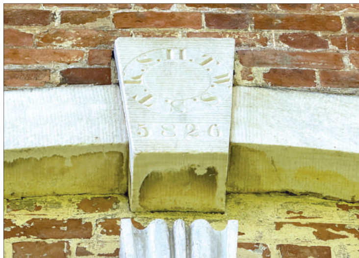
THE KEYSTONE IN the arch above the front doorway bears a Masonic inscription and the Masonic year 5826, which corresponds to 1826, the year the house was built for Barnard Ketcham, an active Mason. The house hosted Masonic rites in the 1800s.
