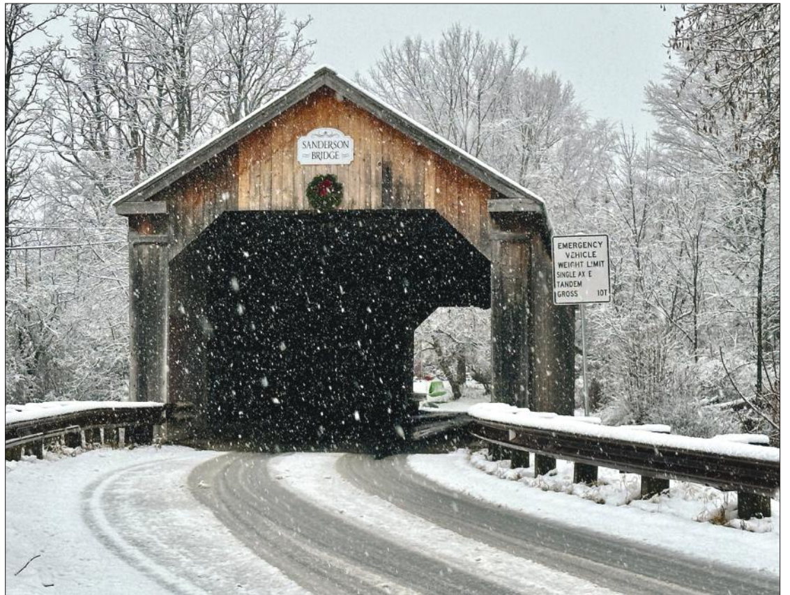
THE SANDERSON BRIDGE on Pearl Street in Brandon straddles the Neshobe River. Once part of the Sanderson farm, the original bridge had deteriorated to the point where it had to be rebuilt in the early 2000s to be usable. The Vermont Covered Bridge Society's Rutland Chapter, headed by Sudbury resident Beth Brown, decorates the bridge (along with all the others in Rutland County) every holiday season.
