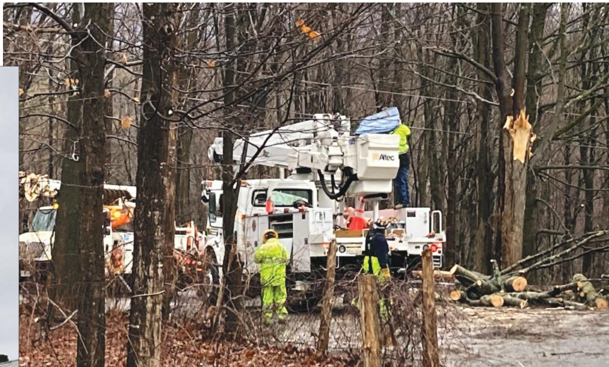
ALYSSA ZOLLMAN OF Prospect Street in Brandon sent us this photo of a GMP repair truck at work restoring power near her home. "Saturday's early morning windstorm caused damage and power outages throughout the region," Alyssa wrote. "Falling trees and branches took down power lines, and in this case, snapped a pole on Prospect St. in Brandon. It was a welcome sight to see this repair crew arrive before dark!"
