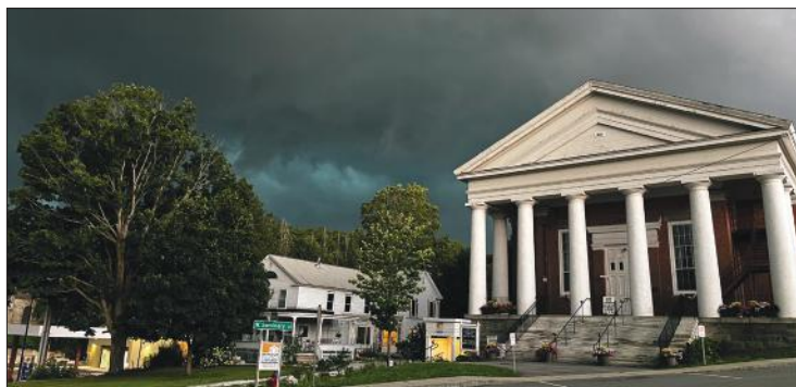
THE MAKINGS OF a tornado swirl above Brandon Town Hall on Thursday, July 13. The winds would knock a stone topper off one of the building's chimneys, damage to the slate roof. Photo by Jeff Sacks
