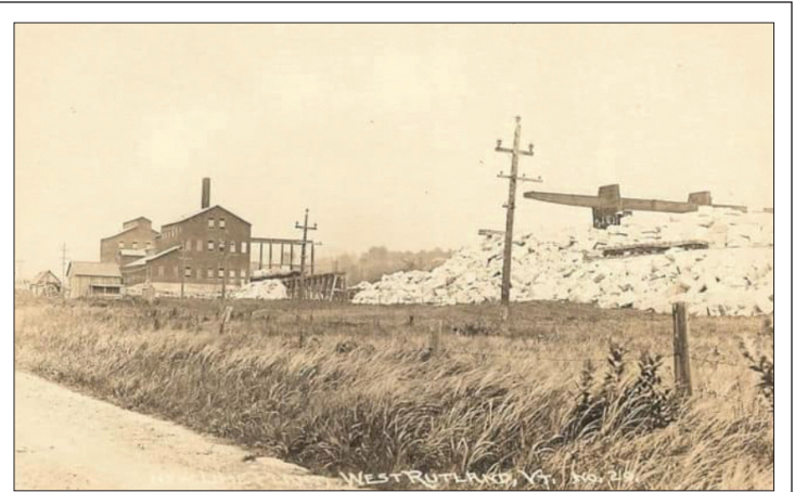
THE WEST RUTLAND Marsh in the early 1900s. Though protected wetlands today, it was the scene of industry and worker housing back in the day. Photos provided.
