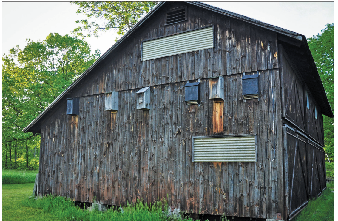
BAT HOUSES ARE a great alternative for bats you need to evict from your home, but they do require some maintenance in the late fall or winter to clean out abandoned wasp nests and repair any leaks. VTF&W photos
