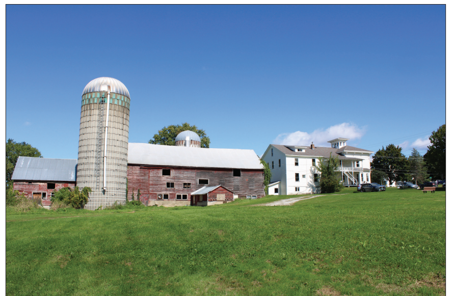
THE PITTSFORD VILLAGE Farm aims to renovate the old farmhouse to hold a community center and an early childhood education center as well as apartments.
